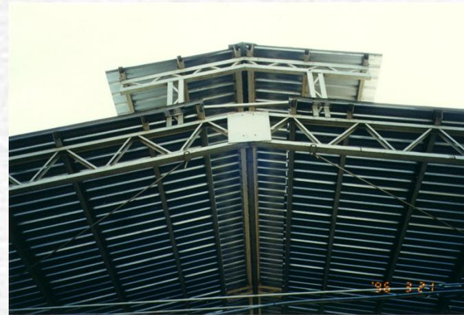
$\Delta T$ ,  $\Delta h$  and ratio of opening area are critical factors in natural ventilation
