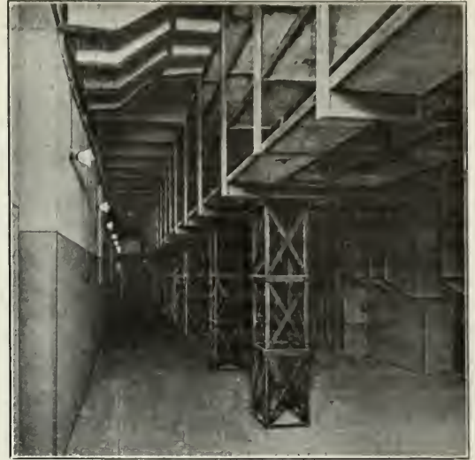
FIG. 14.—FIRST FLOOR OF SWITCH-HOUSE; 10,000-VOLT BUS-BARS.
