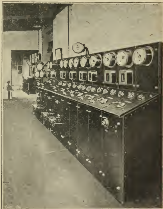
REMOTE CONTROL BOARD FOR THE E.H.T. SWITCHGEAR.
