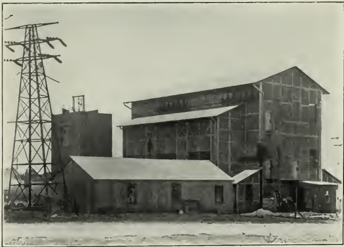
FIG. 23.—DISTRIBUTION STATION AT BANTJES FED FROM 40,000-VOLT OVERHEAD LINE.
