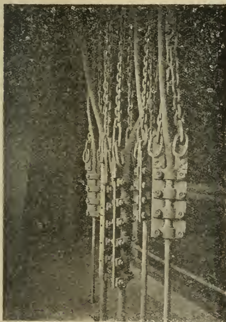
FIG. 8.—SINGLE SUSPENDERS OF THE CLAMP TYPE, SUPPORTING PAPER-LEAD-COVERED AND WIRE-ARMOURD CABLES, AT THE PRETORIA PIT
