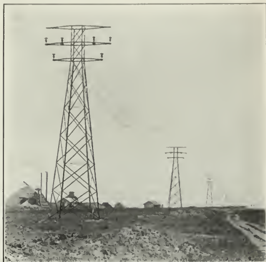
FIG. 21.—OVERHEAD LINE AT 10,000 VOLTS.
