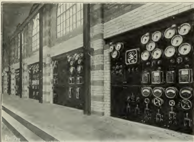
FIG. 1.—THREE-PHASE E.H.T. SWITCHBOARD, NEW POWER STATION, STOKE-ON-TRENT.
