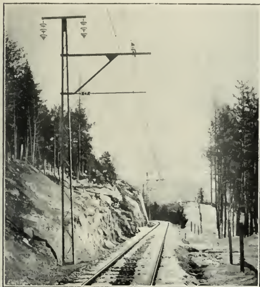
TYPICAL VIEW, MITTENWALD RAILWAY, SHOWING POWER TRANSMISSION LINE.
