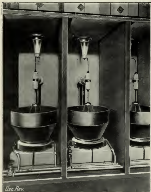
FIG. 16.—WATER-JET DISCHARGERS FOR 50,000-VOLT LINES.
