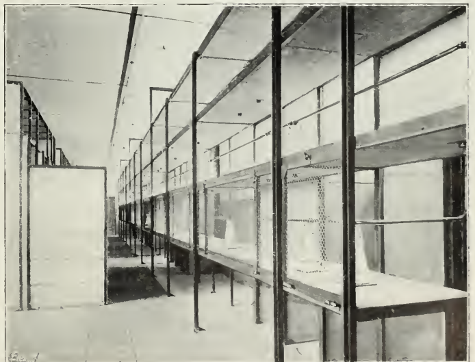
FIG. 15.—SECOND FLOOR OF SWITCH-HOUSE; 50,000-VOLT BUS-BARS.
