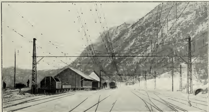
ARRANGEMENT OF CONTACT LINE, SAAHEIM STATION: RJKUAN RAILWAY.
