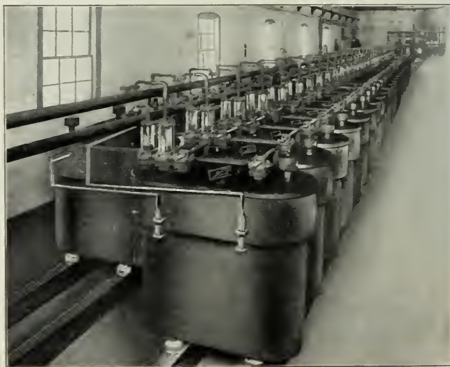
AN INSTALLATION OF OVAL TYPE I.O.C. GENERATORS.
