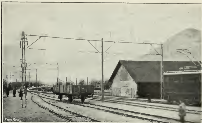
CONTACT LINE AT SHUNTING STATION, MITTENWALD RAILWAY.
