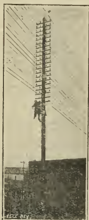
FIG. 2.—CREOSOTED POLE, DATED 1900, CARRYING 68 WIRES: PROBABLE LIFE, 20 YEARS LONGER.
