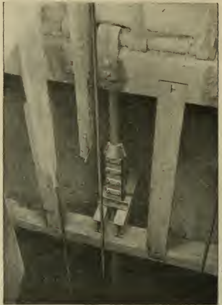
FIG. 5.—SITTING TYPE OF WOODEN CLEAT FOR SHAFT SUSPENSION, RESTING ON EXISTING BUNTONS.
