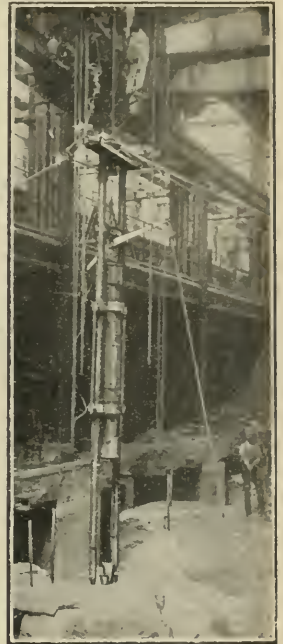
CONCRETE-BREAKER AT WORK AT BANKSIDE.
