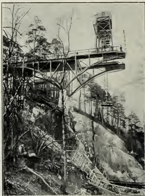
FIG. 11.—CANTILEVER GANTRY CRANE, 42 TONS.
