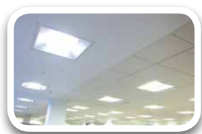
Recessed type LED lighting panel 嵌入式LED燈盤
