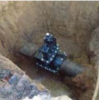
new valves in existing mains. Alternately, a solid sleeve can be used to install a new valve in an existing main. With this method, the valve should be held firmly in place in the line by using a filler piece of pipe to fill the gap
