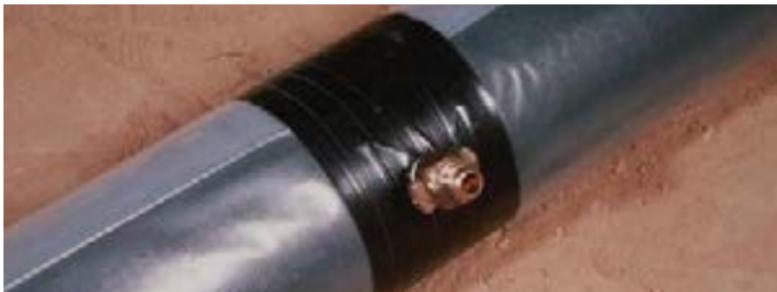
The preferred and recommended method of making direct service taps on polyethylene-encased pipe consists of applying two or three wraps of polyethylene adhesive tape completely around the pipe to cover the area where the tapping machine and chain will be mounted. This method minimizes possible damage to the polyethylene during the direct-tapping procedure. After the tapping machine is mounted, the corporation stop is installed directly through the tape and polyethylene as shown.
