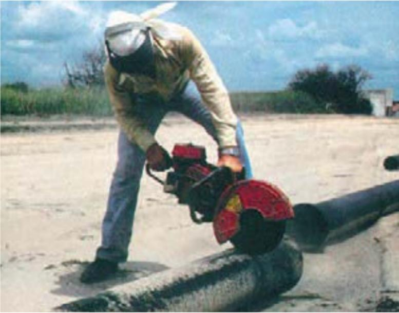
**3.11 Cutting Pipe:** Ductile Iron Pipe can be cut using an abrasive cut-off saw, a rotary wheel cutter, a guillotine pipe saw, a chain saw specifically made to cut Ductile Iron Pipe, or a milling wheel saw. The pipe can also be cut with an oxyacetylene torch if recommended by the pipe manufacturer.
