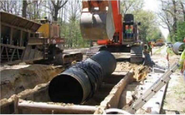
**1.4 Slings:** A variety of slings are available for handling pipe. Nylon slings, with an appropriate lifting capacity, are particularly well-suited for lifting Ductile Iron Pipe and appurtenances.
