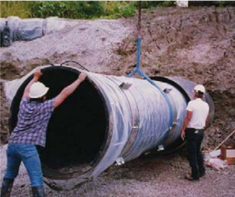
Where casing is required, the Ductile Iron Pipe is either pushed or pulled through the previously
