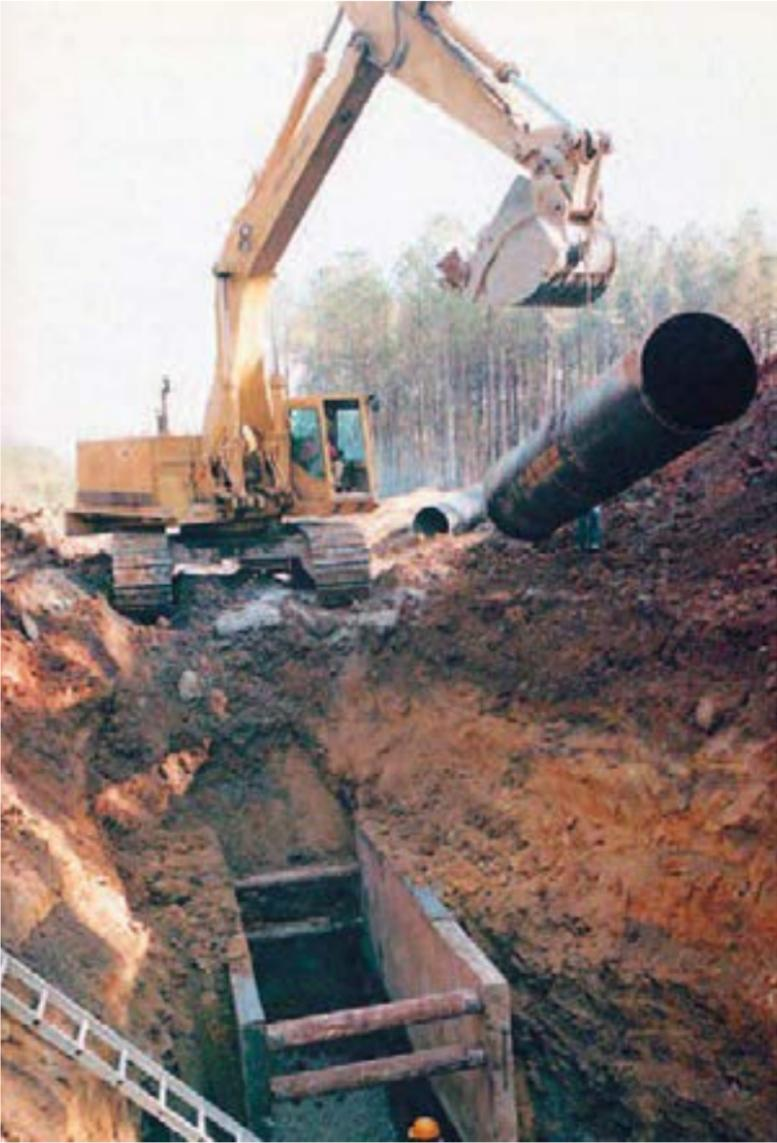
**3.4 Direction of Bells:** Although it is common practice to lay pipe with the bells facing the direction in which work is progressing, it is not mandatory. When the main is being laid downhill, for example, the pipes are occasionally laid with the bells facing uphill for ease of installation. The direction of the bells is not functionally related to the direction of flow within the main. See Section 2.8, Bell Holes, for additional comments relating to direction of bells.
