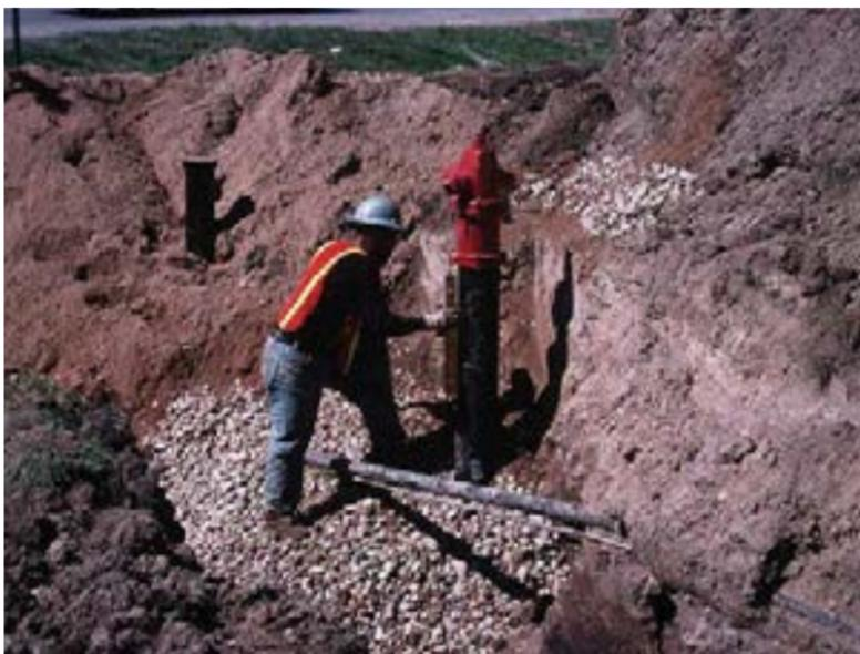
Most hydrants have a grade-line marking and should be ordered for the proper depth of pipe cover so that the hose and pumper nozzles will be at the correct height. The connecting line to the supply main should be no less than 6-inches in diameter. Refer to AWWA Manual M-17 for proper fire hydrant installation.
